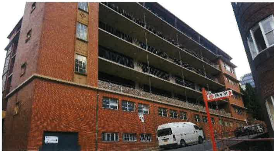
Figure – Looking north west from the corner of William and Blue Streets towards the eastern elevation of the building at the Shore School
