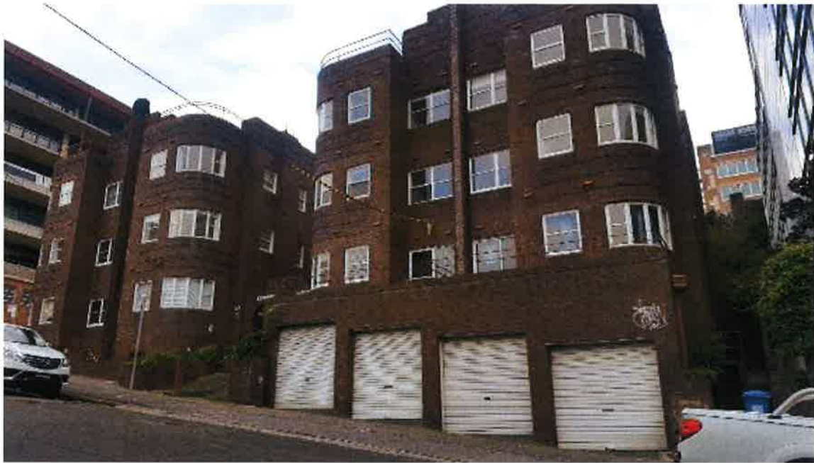
Figure – Looking north from Blue Street towards the subject site (No's 2 and 4 Blue Street)
